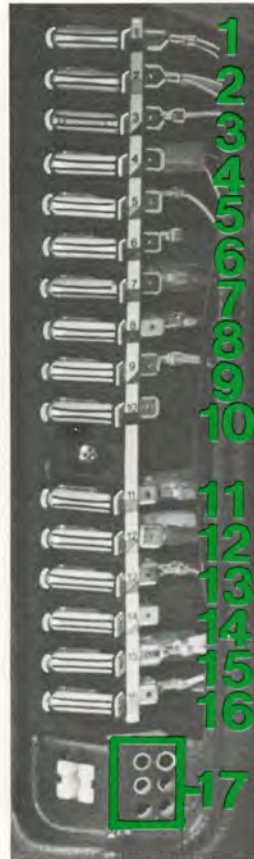
17 Fuse storage, spare
